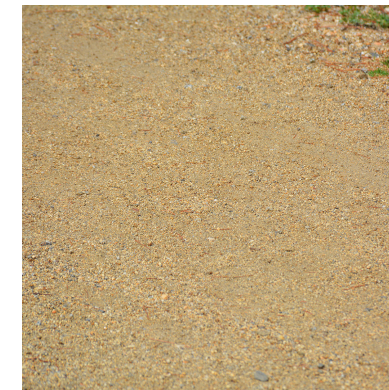
COMPACTED GRANITIC SAND PATH
