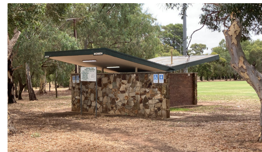
Park 17 existing toilet facility at corner of Greenhill and Glen Osmond Road.
